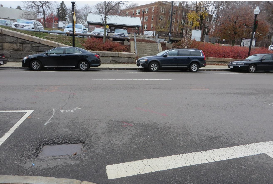
The steps at the Commuter Rail Station do not connect to a pedestrian crossing on Belgrade Avenue.
