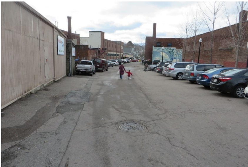
The private parking lot between South and Corinth Streets (Taft Court/List Place) lacks adequate pedestrian accommodations.
