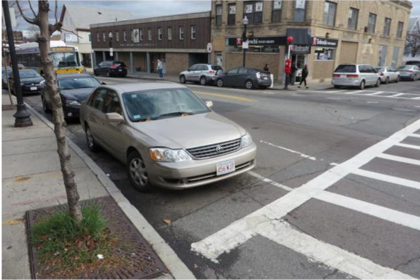
Cars encroach on the crosswalk at Washington/South/Basile Streets, which also lacks a curb cut.
