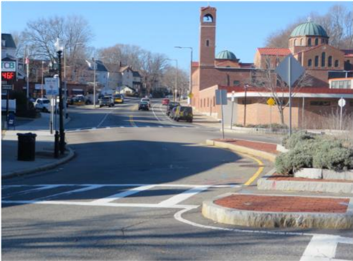
The intersection of Belgrade Avenue at Corinth and Roberts Streets is confusing to navigate, with wide travel lanes and turning radii encouraging high traffic speeds.
